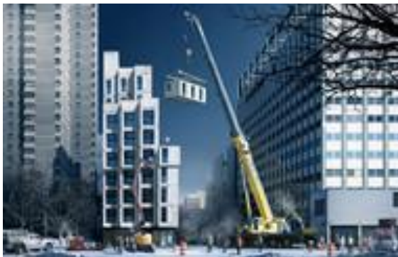
A computer visualization of the erection of the micro-apartment development. Each apartment will be prefabricated in a factory in Brooklyn, then craned into place almost fully finished. The process is intended to improve construction quality and save money. Source: nARCHITECTS /Museum of the City of New York via Bloomberg
